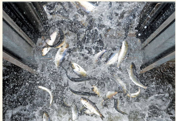
Photo above: River herring pour out of the fish elevator at the Benton Falls Dam. A fish elevator, or lift , carries fish over a barrier (the dam). Fish swim into a collection area at the base of the dam. When enough fish accumulate there, they are moved into an “elevator” compartment that carries them into a flume that empties into the river, above the dam. At left: An Osprey catches a river herring along the Sebasticook River.
