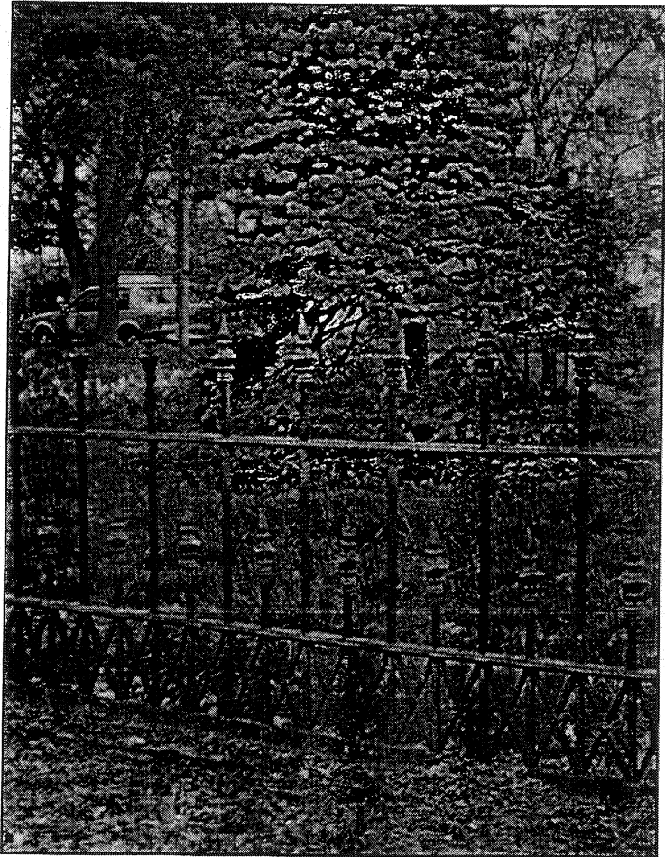
Castings were made to replace a limited number of lost finials along the perimeter fence of Lafayette Square, St. Louis, Missouri. (author, 1994)
