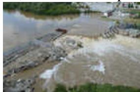
High water volumes from Tropical Storm Irene stalled progress at a work site at the Worumbo Dam in Lisbon Falls earlier this week. This photo, taken from Ed Friedman's helicopter Tuesday, shows the water volume and the temporary coffer dam, left, installed for the reconstruction project. Work on the project resumed on Wednesday, according to Miller Hydro officials.
