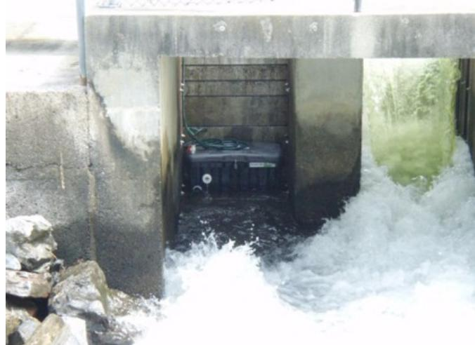
**Type:** Partial height ramp trap, gravity supply
