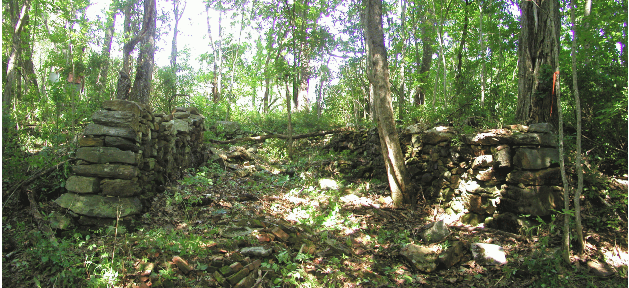
Figure 11. Panoramic view, looking eastward into the open end of the foundation of the dwelling structure at ME 049-009. Note pile of chimney brick left foreground from a collapsed chimney.
