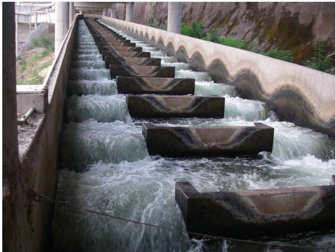
Fig. 3. Fish ladder at the Lower Granite Dam, Snake River, Washington. Ladders such as this allow passage at dams that would otherwise extirpate upriver runs but can delay upriver migration. Photo credit: Thomas P. Quinn.
