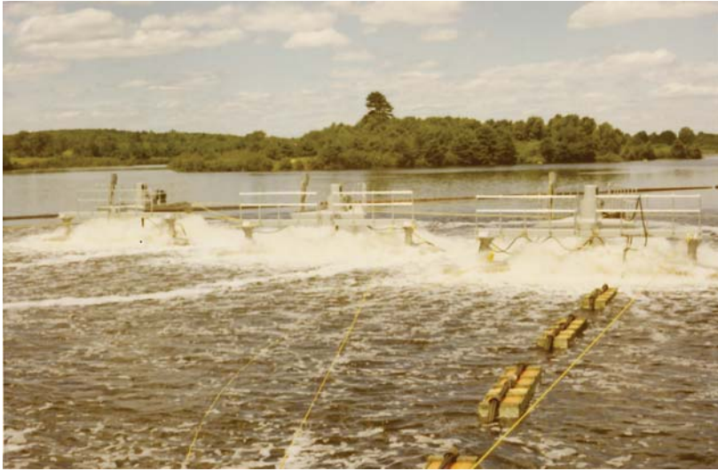
Figure 5: Using mechanical aerators on the Androscoggin's Gulf Island Pond, Lawrance attempted to recreate the natural oxygenation that the river's many impounded falls had once provided. Credit: Androscoggin River Studies Annual Report 1969, 102. Walter A. Lawrance papers. Edmund S. Muskie Archives and Special Collections Library, Bates College.
